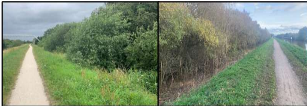
Photos 5/6: Before bushing works between Burton Waters and the A57 on Fosdyke (left), and after completion of works (right).
